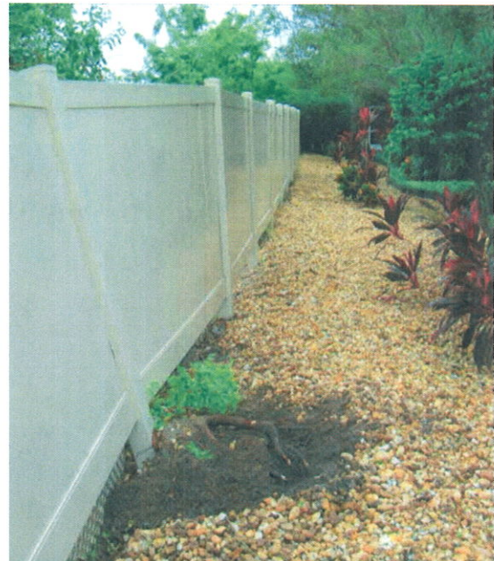
Looking east along the south bank of Channel 1 (west of 66th Street North) behind the condominium fence
