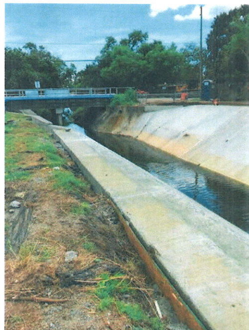
Looking east – transition to exiting channel
