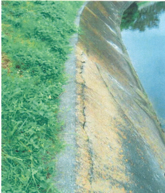
Channel 1 – Looking west along the south bank of Channel 1 (west of 66th Street North)
